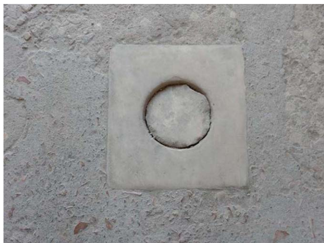
Figure 11. Pompeii, Domus Sirico (VII 1, 47), detail of inspection hole with marble cover (photo by the author, published with permission of the Ministero della Cultura - Parco Archeologico di Pompei).
